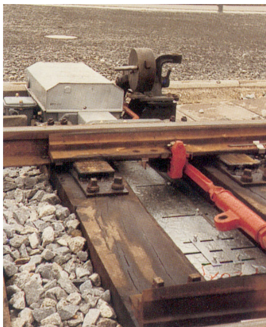
Point interlocking heating system placed underneath the switch rodding and embedded on ballast
