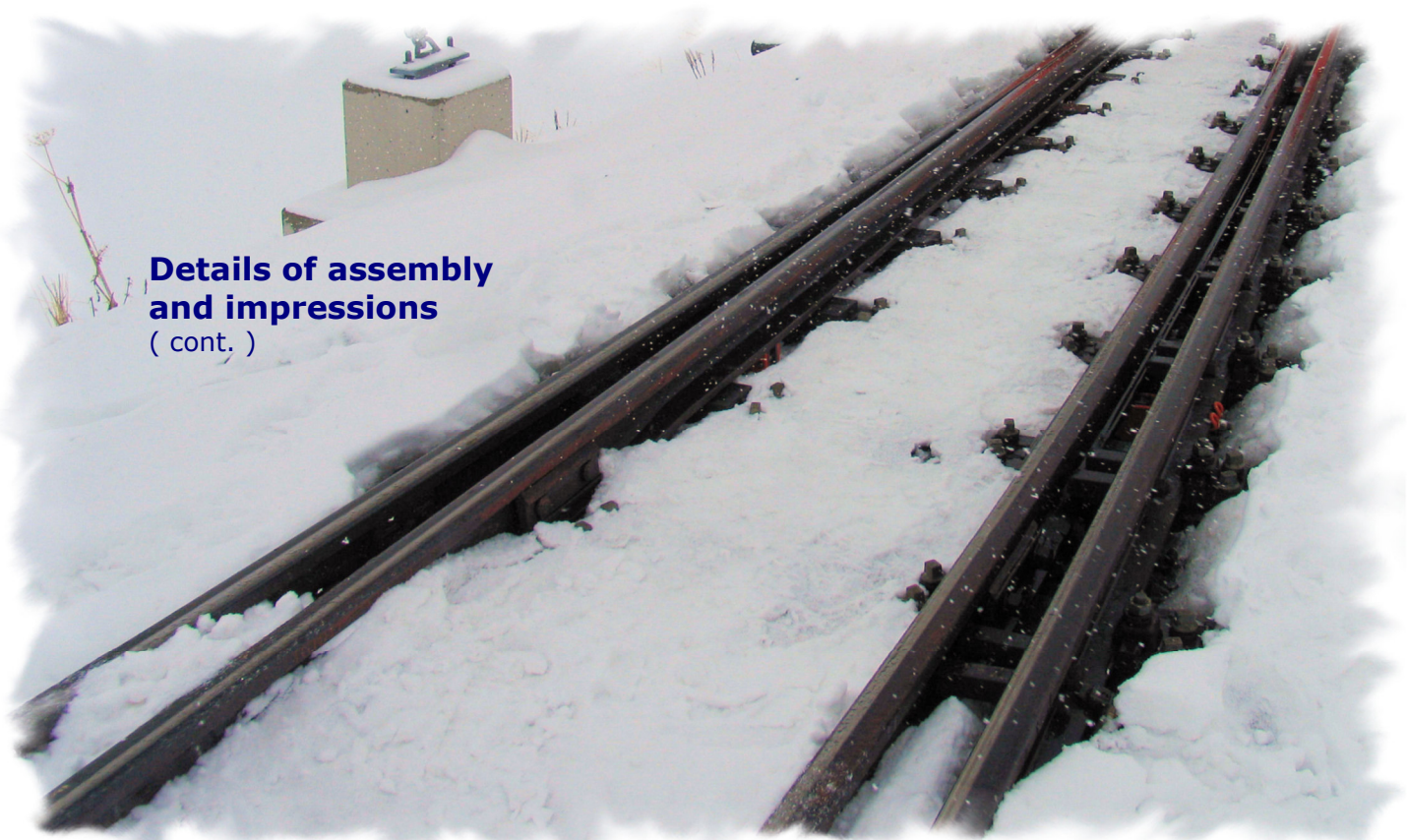
Heating elements of Backer ELC at Oberalp-pass at the Matterhorn Gotthard Railway
