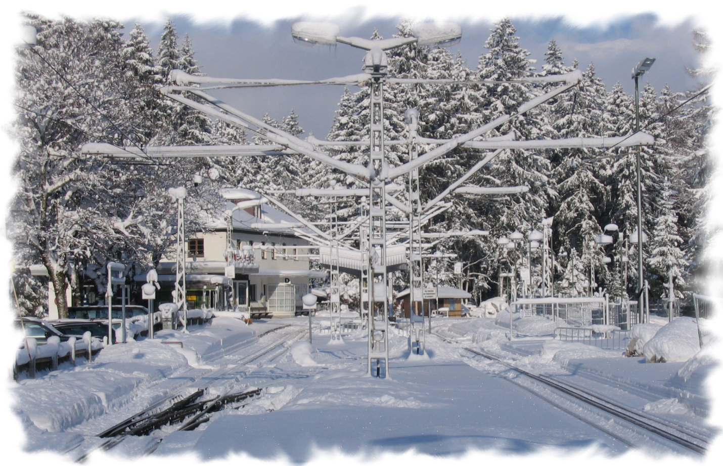
Backer Wolff point heating system at Eibsee station at Germany's highest mountain the Zugspitze
