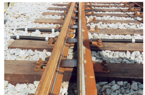
Switch blade gliding over connecting head; bottom view
